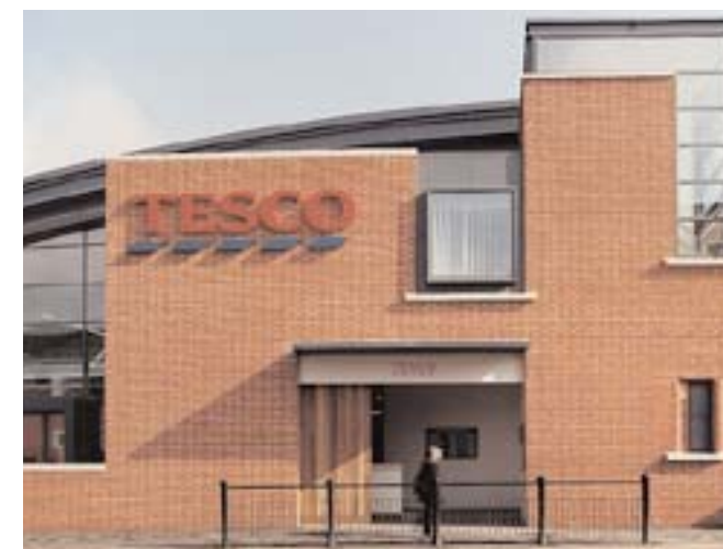
The frontage to Corve Street is composed of hand-made local brick.
