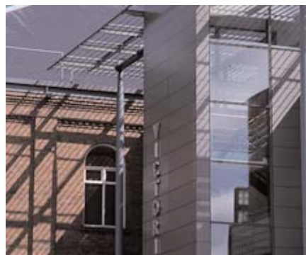
The junction between old and new is handled sensitively and with a light touch.
