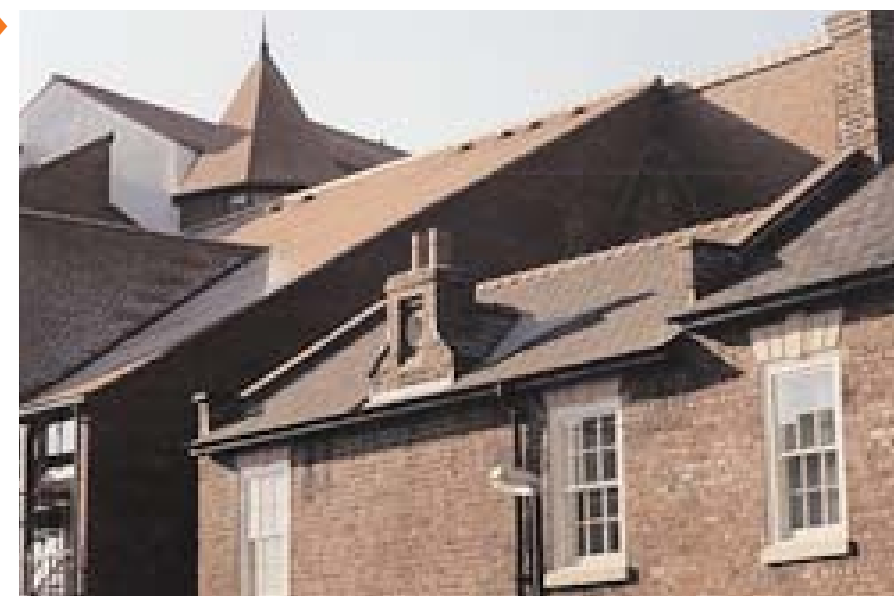
Another listed building forms the corner of the site on the Bars.
