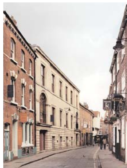
At the rear of the site, on Little Stonegate, a former chapel has been carefully restored.
