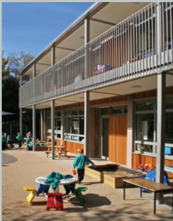
Burnham Copse Primary School, by Hampshire County Council © Dan Keeler
