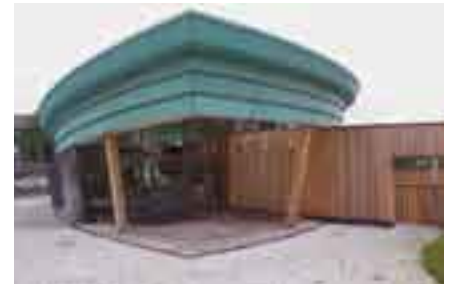
Above: The approach to the front door.
