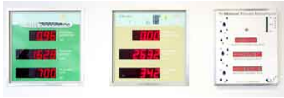
Above: Inside the building, three digital panels indicate the building's use of power and water.
