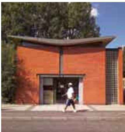
Above: The gull-wing roof gives the front of the surgery its distinctive appearance.
