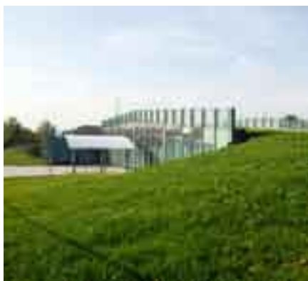
Above: The majority of the building is set beneath a grass roof.
