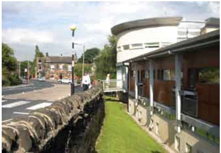
Above: Road-side approach to the Idle Medical Centre.
