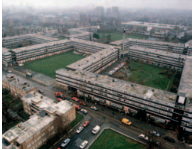
Aerial view: Holly Street snake blocks before demolition
