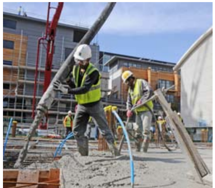
Green concrete at One Brighton by Crest Nicholson BioRegional Quintain – 100% recycle aggregate and 50% cement replacement reduces the embodied carbon by a third
