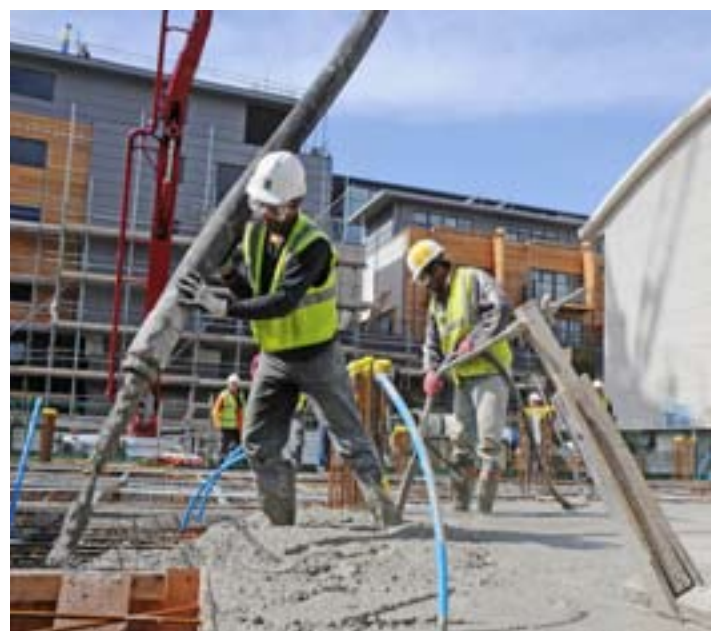
Green concrete at One Brighton by Crest Nicholson BioRegional Quintain – 100% recycle aggregate and 50% cement replacement reduces the embodied carbon by a third
