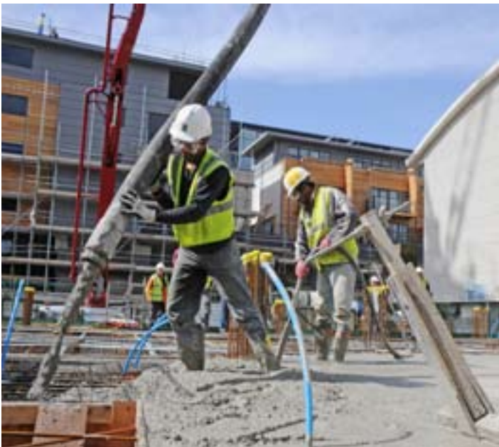
Green concrete at One Brighton by Crest Nicholson BioRegional Quintain – 100% recycle aggregate and 50% cement replacement reduces the embodied carbon by a third
