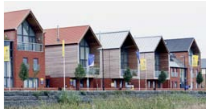
Aspect Upton Way, Northampton. This award-winning new development shows what an eco-town could look like. Built to EcoHomes Excellent standard, it incorporates glazed passive solar design and photovoltaic panels on the roof.
