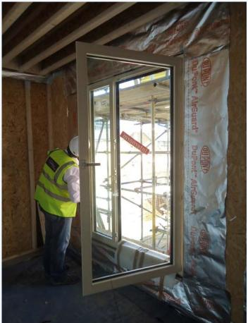
In response to these creative challenges, Cartwight Pickard designed two of the buildings to incorporate a superstructure of Structural Insulated Panels (SIPs)<sup>2</sup>. The other two buildings used a concrete frame with SIP panel and brick cladding.
